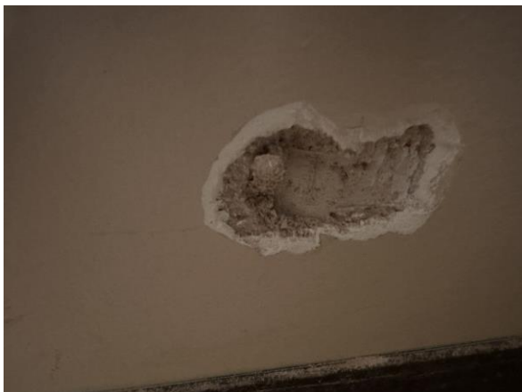
Photo 17 HA-22: Hard plaster material skim coat over cement walls
