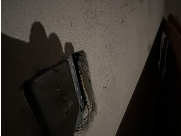
Photo 13 HA-17: Beige cement wall coating
