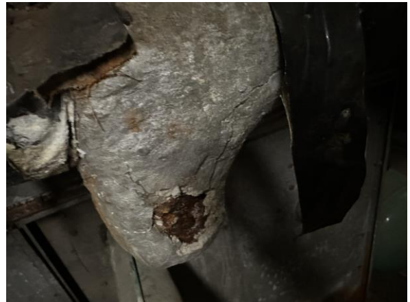
Photo 10 HA-11: Grey and white plaster patching at connection points
