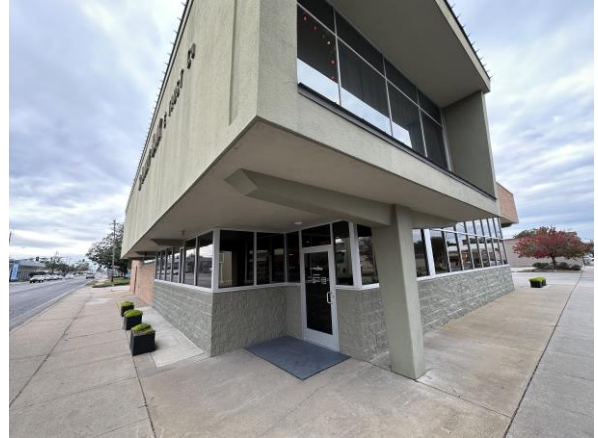
Photo 14 HA-19: Exterior stucco
