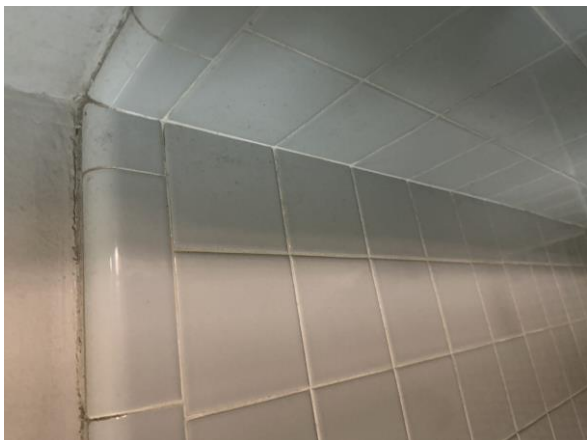
Photo 5 HA-5: 3.5"x3.5" Green ceramic wall tile with grout
