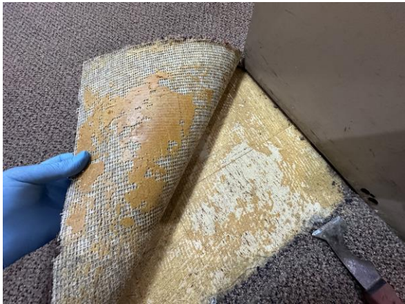
Photo 3 HA-3: 9"x9" White and beige floor tile with black mastic
