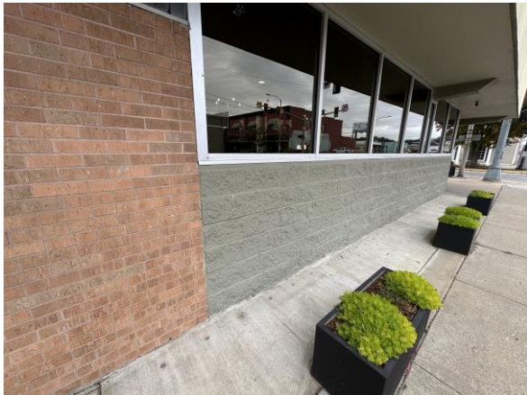
Photo 15 HA-20: CMU blacks and mortar
