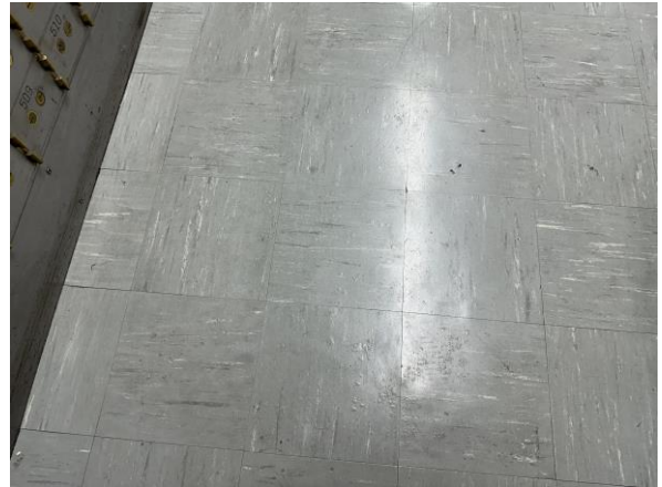
Photo 8 HA-9: 9"x9" Grey and white floor tile with black mastic
