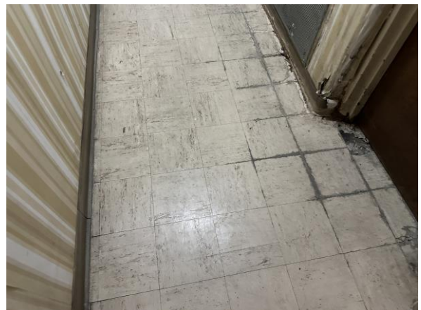
Photo 6 HA-7: 4" Brown cove base with mastic
